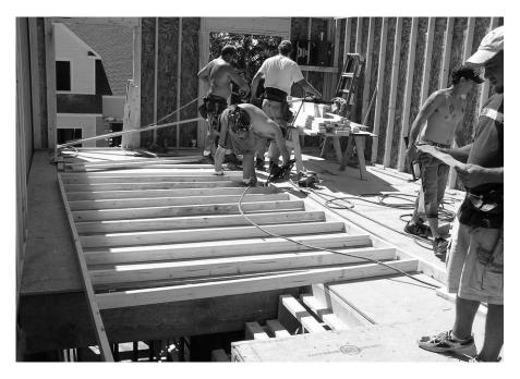
Figure 5-10: "Stick-Build" Framing Process
