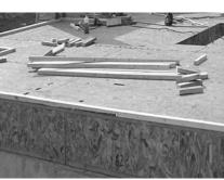
Install the sole plates for the first floor wall panels
