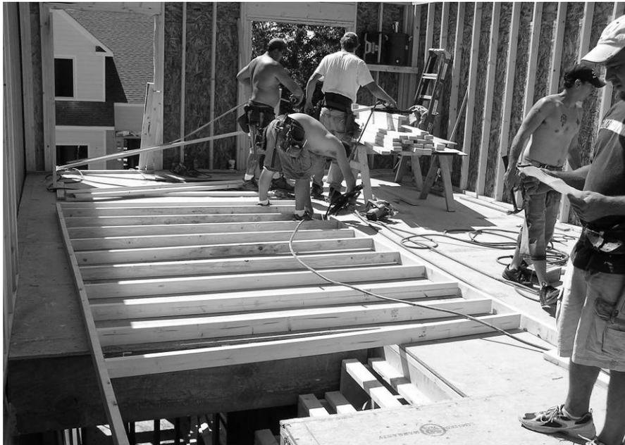
**Figure 5-10: “Stick-Build” Framing Process**
