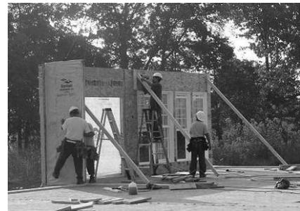
Install other wall panels on the first floor piece by piece and nail or screw them together
