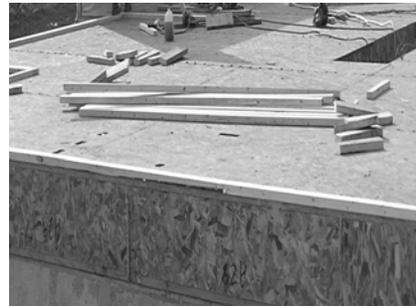
Apply sealant on the sole plate
