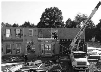
Install the roof trusses
