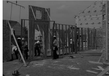
Install the top plates on interior walls
